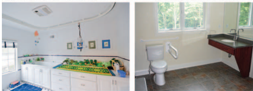
Top: no step covered entry. Bottom left: raised tub and changing counter with ceiling-mounted lift system. Bottom right: Accessible commode and roll-under sink.
